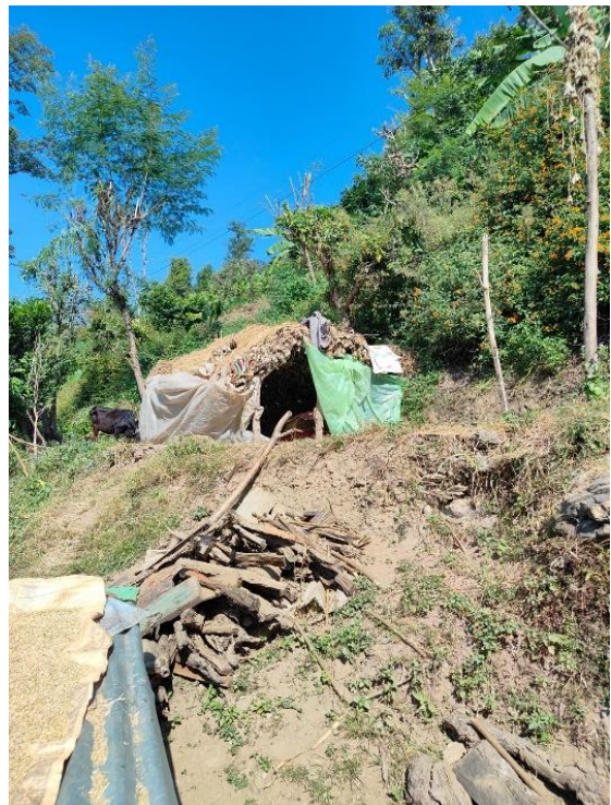
Figure 13. A temporary shelter built after the earthquake in Bheri Municipality Ward No. 3
